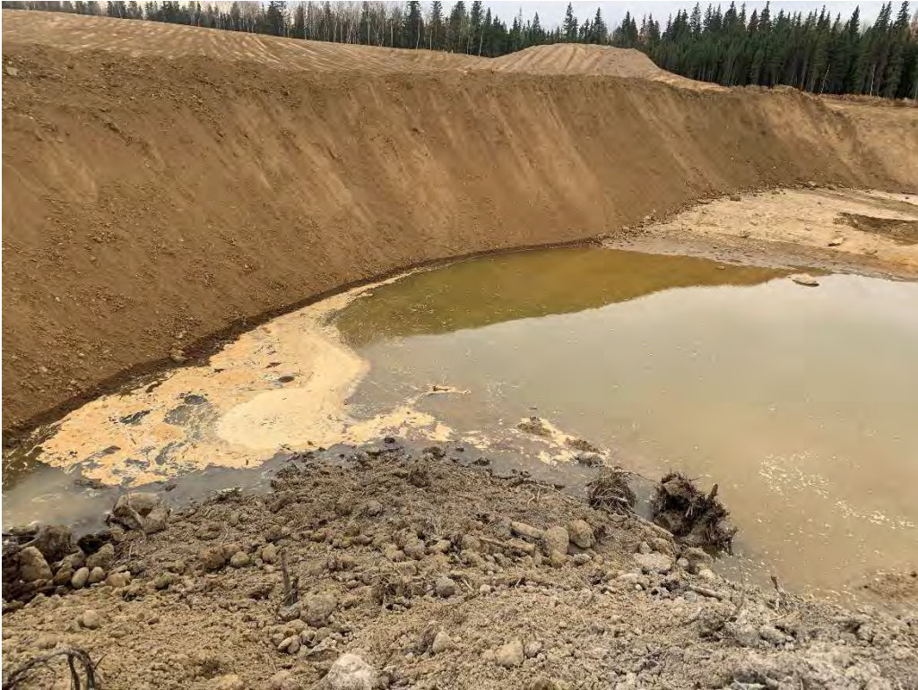
Photo 4: Photo taken looking North of the backfill filling in the waterbody.
