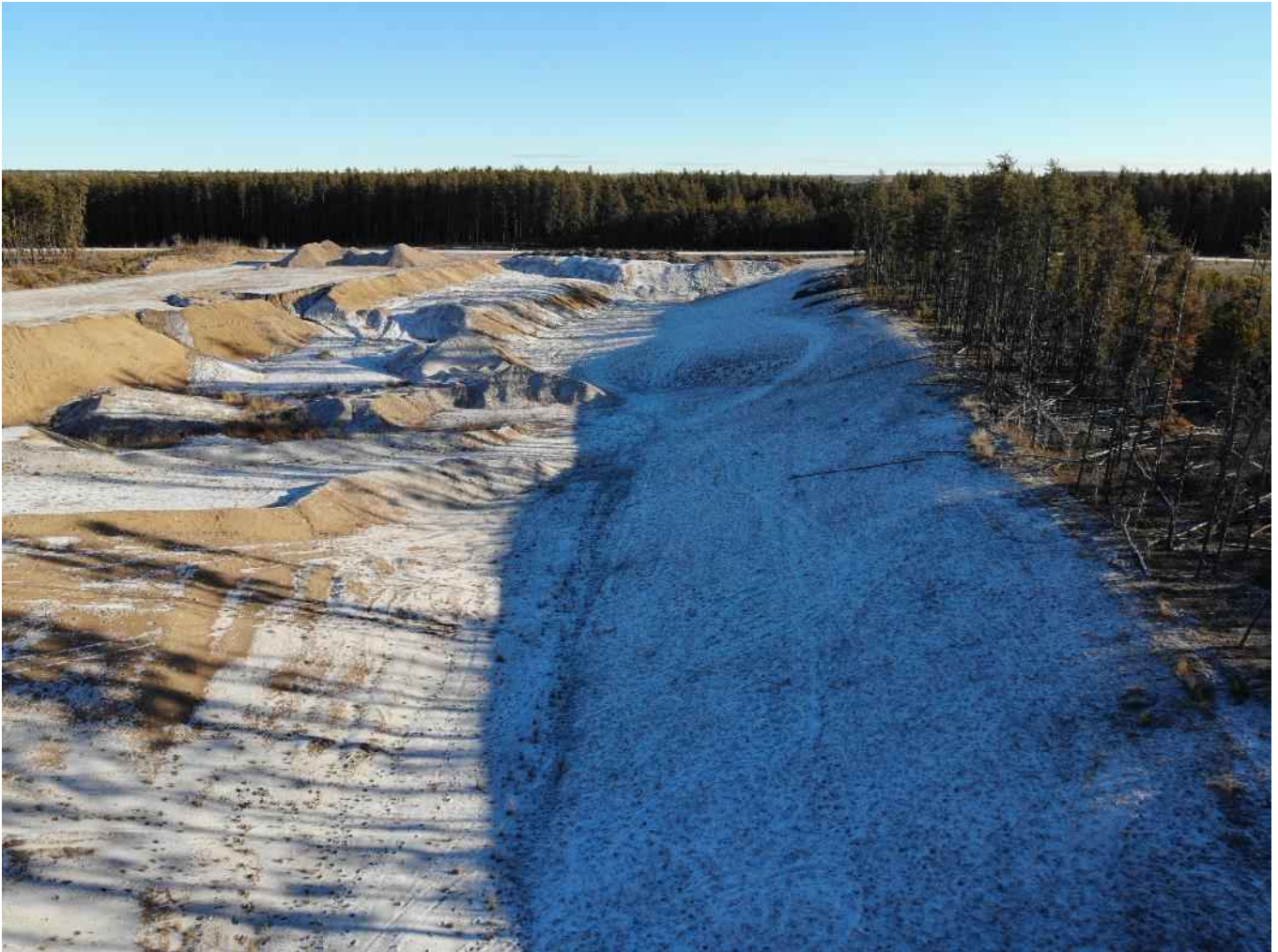
Drone overview looking east along the south boundary of the Pit. The image shows the approximate slope of the south boundary of the Pit as well as the condition of the excavation in the south part of the Pit.
