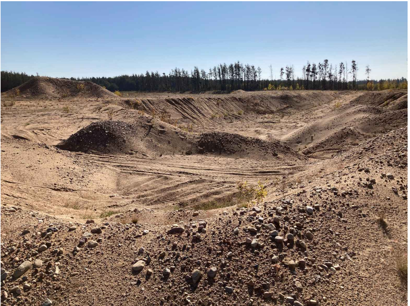
The excavation in the middle part of the lease, as observed September 22, 2023, looking southeast.
